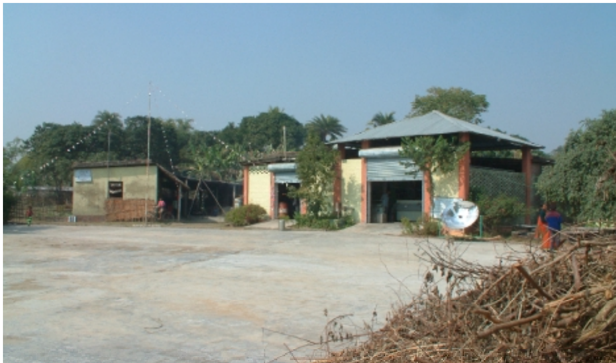
EmPower Partnership Power Plant and Micro-industries in Baharbari, Bihar.
