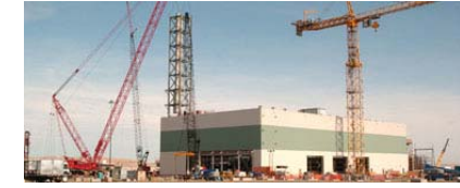
Waste Treatment Plant Construction, Hanford, Washington, 2008
