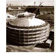
Tank Construction, Savannah River, South Carolina, 1963
